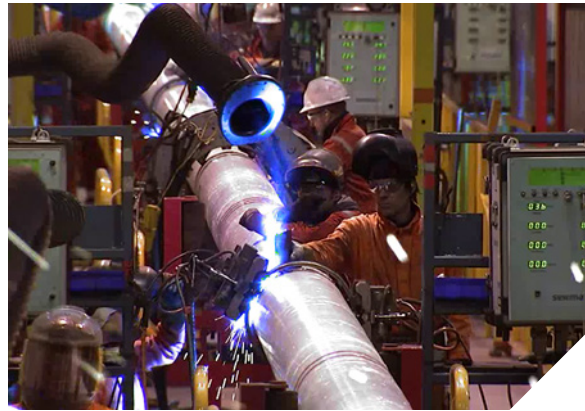
Welding at spoolbase
